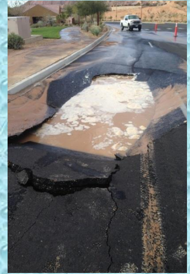
Pipe Break Falcon Ridge Parkway
