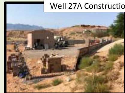
Well 27A Construction
