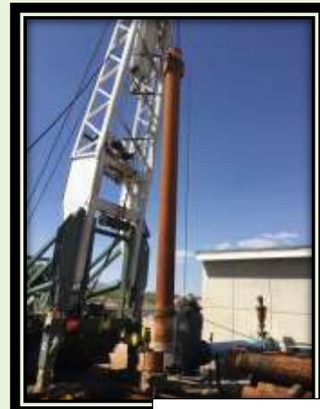
Well 31 Pump Replacement
