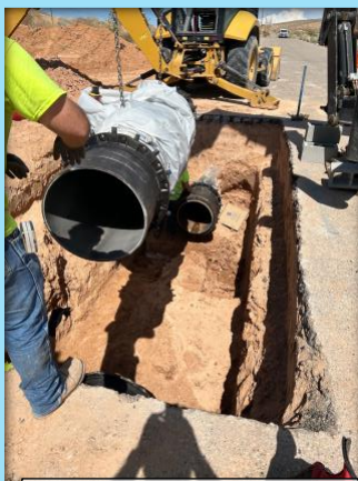
Another Break Repair
